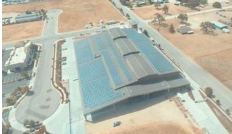
REC Solar completes solar project for San Antonio Winery's Paso Robles production facility August 22, 2017 In "Business"
